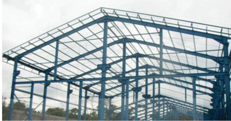
**Gambar 5.30** Rangka Atap Baja Konvensional
